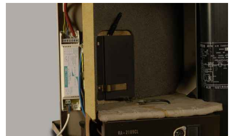
9 Position sensor in supply air stream (example)
