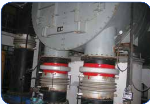
DN700 Sialex® Ring on condenser unit
