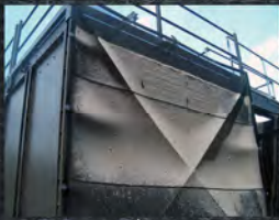
Willoworeek Church Martley Cooling Tower
